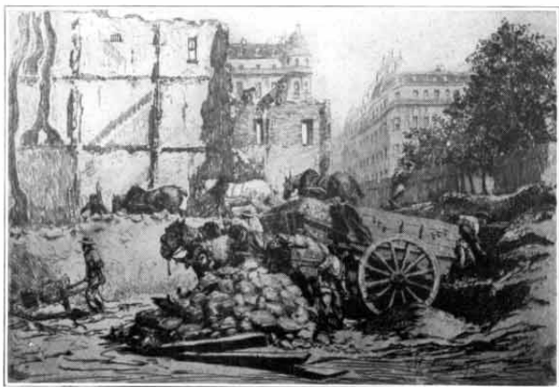
EXCAVATION G. W. Chandler
